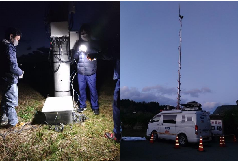
Leveraging SpaceX's Starlink in place of the severed fiber-optic cables to restore base stations
